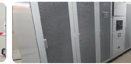
Thailand Project B, TikTok Project Data Centre Power Backup Project 512V 210Ah
