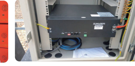
Indonesia Project Telecom Power Backup 48V 100Ah
