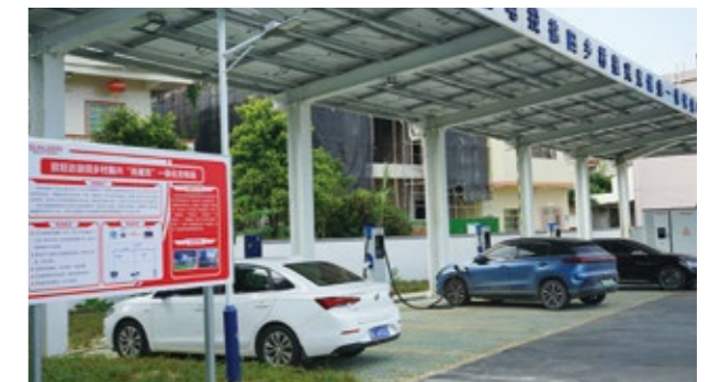
The First Rural Revitalization Solar-Energy Storage Charging Project in Xutian Village, Huizhou
