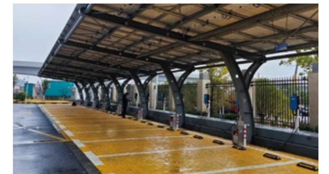
Nanchang Photovoltaic-Storage-Charging-Inspection Project
